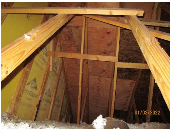
Attic Framing/Sheathing:
