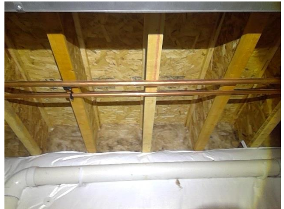
Under Floor Framing & Support:
