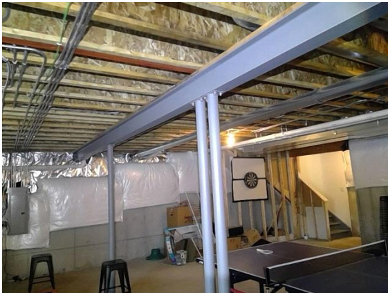
Under Floor Framing & Support:
